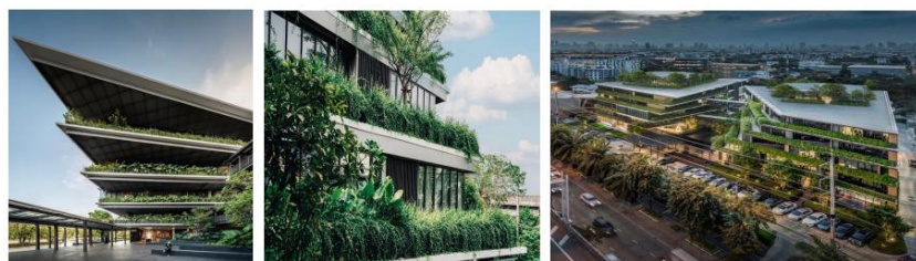
Figure 19: Proposed new acquisition – 111 Praditmanutham office building
