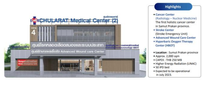
Figure 7: Chularat Medical Center (opening July 2023)
