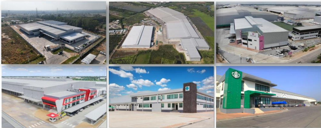
Figure 19: Warehouse portfolio (existing assets)
