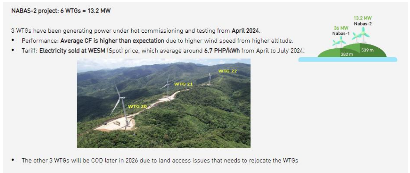
Fig 4. Nabas-2 Project: 3 WTGs is under hot commissioning and testing and SCOD for remaining 3 is scheduled for 2026
